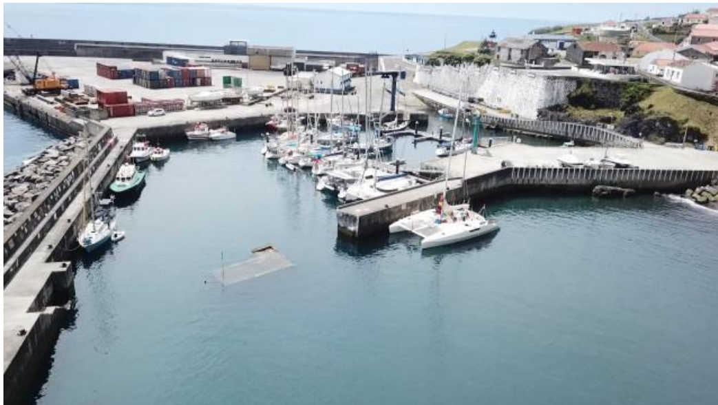
Flores harbour, as seen by the drone. You can make out the dangerous lump of jetty right in the entrance
