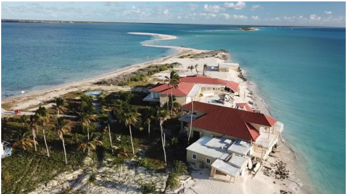
Hurricane-induced breach into the main lagoon in Barbuda
