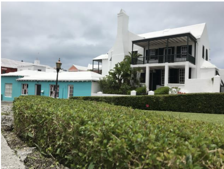
Bermudan roofs – universally whitewashed, and with a unique rain-catching gutter which funnels all the rainwater into storage
